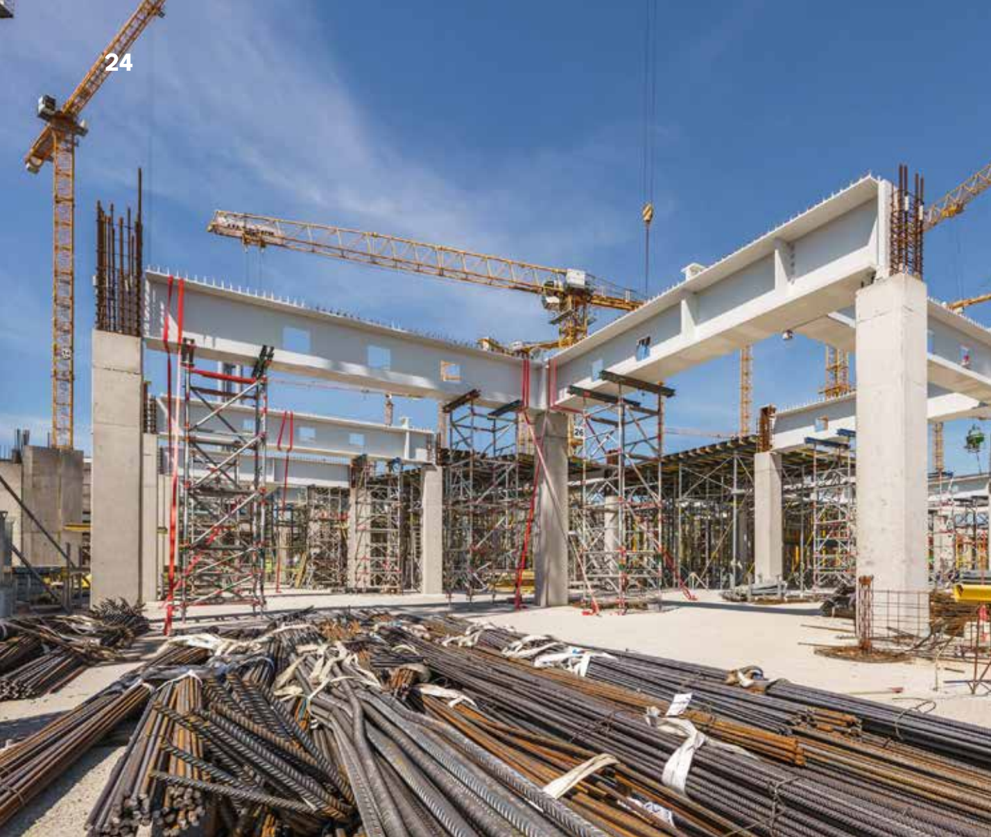
There are wide-span beams above the mall and complex areas, as well as heavily loaded beam grids in the cruise terminal area
