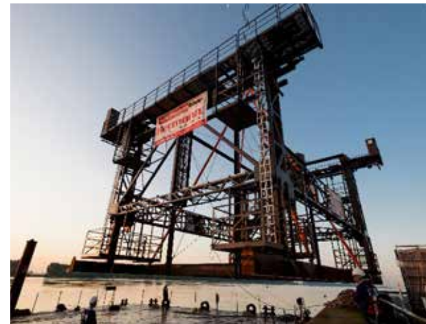
The suspension railway unit with the pre-assembled bogie is loaded onto a pontoon
