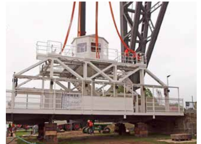
Before the platform can be connected to the carriage, it must first be positioned at the correct height and angle on the wooden stacks
